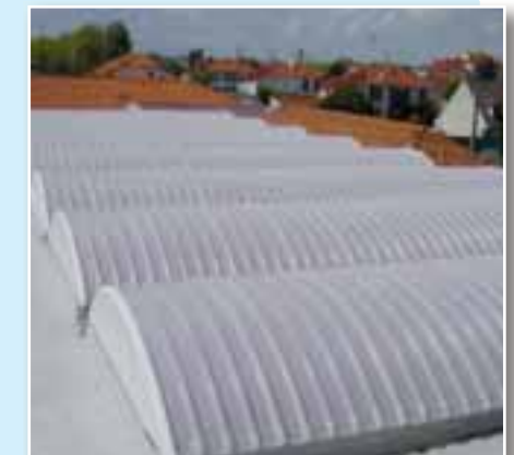
Refurbishment - Colombes - FR
