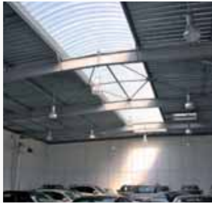
New building project - Paris - FR
