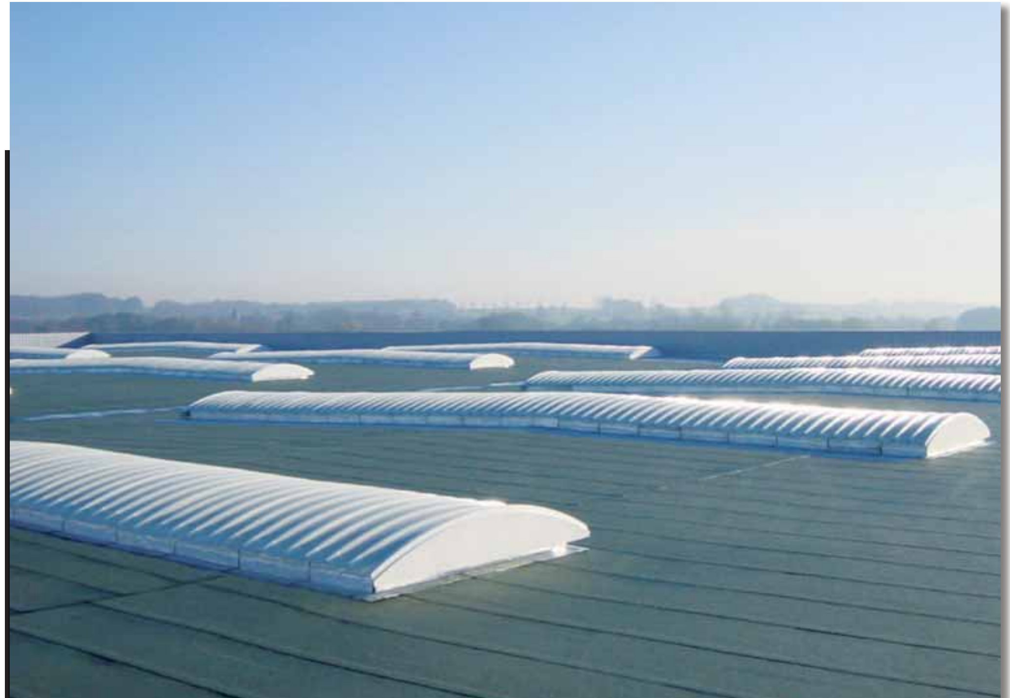
Refurbishment - Warsaw - PL
